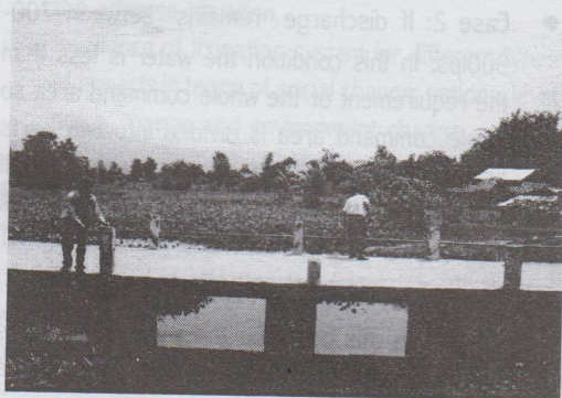
Photo 2: Wetland area at the headworks
